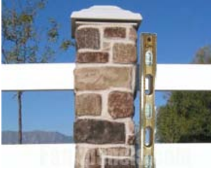
7. Level post before concrete sets
