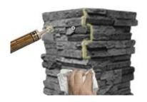
**8.** Before the texture caulk dries be sure to use a damp rag to wipe off any excess caulk that may have squeezed out for between the joint between the two column panels. Use the textured caulk to conceal the screw heads as well.
