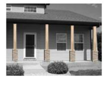
9. Now you can start the next row up if you are installing multiple rows of Faux Column Wraps. Repeat steps 4-9 for the next row of column panels to be installed. Note: The column panels were designed to butt up to each other bottom to top. This joint should also be caulked to insure a tight seal that has a seamless look.
