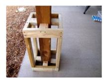
3. Then apply the exterior grade plywood to the wood sub frame to serve as the surface for attaching the Faux Column Wrap panels. Dry fit the Faux Column Wrap panels onto the structure to ensure proper sizing.
