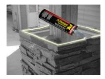
12. Apply glue to the tops of the tops of the Column Wraps and to the wood sub-structure to secure the Column Cap in place. Glue the two halves of the cap together and set it in place, pressing down firmly. Use screws to hold the two halves of the cap together and also to hold the cap to the panels and sub-structure.
