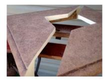
10. Cut the Column Cap into two halves. The cut is made along the diagonal in order to help hide the seam by following the original creases of the cap. Then make a cut out in each of the two cap halves to allow them to fit around the existing porch support post.
