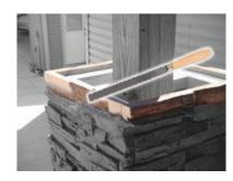
11. Prepare the Faux Column Wrap to accept the Column Cap over it. To obtain a good tight fit of the two halves of the column cap some of the top 1.5" - 2" of the panels had to have some of the stone protrusions shaved down slightly.
