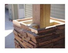
5. Apply the Faux Column Wrap to the plywood. Use a slight twisting motion to help insure a good contact with the glue/adhesive, and the plywood. The PL® Premium Advanced 3X Construction Adhesive will help to hold the individual column panels in place on the plywood and give you some working time to put the other column panels up.
